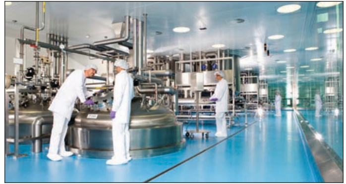
Test runs under production conditions.
