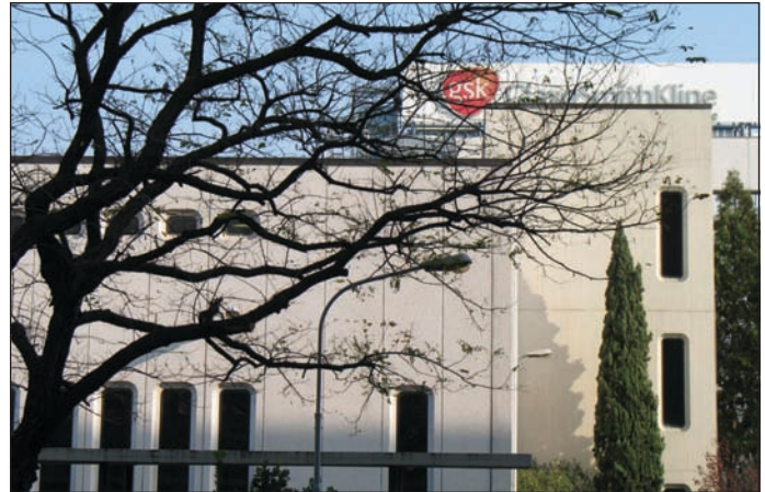
Aseptic powder filling facility.
